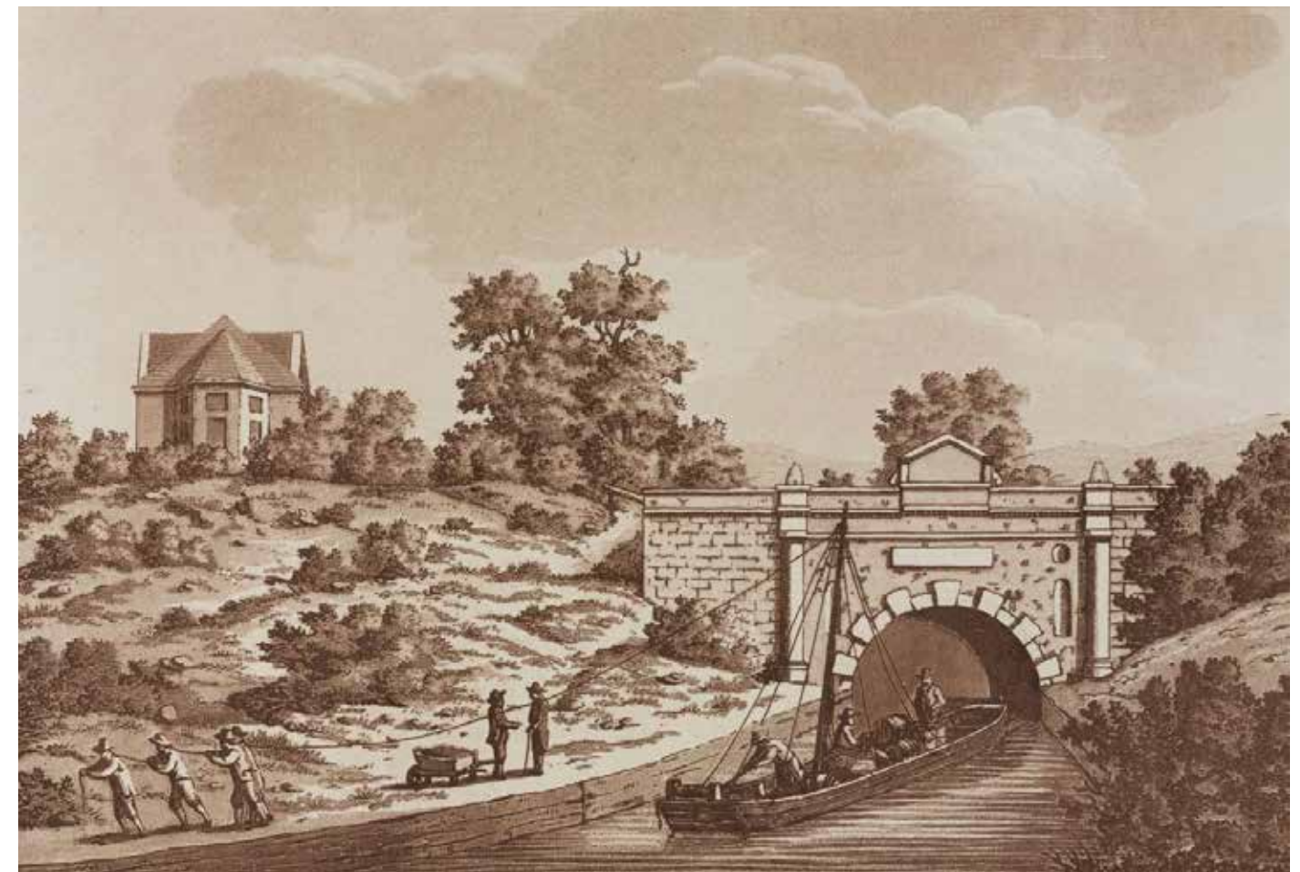
Coates entrance to the Sapperton tunnel (CC SA 1.0)
